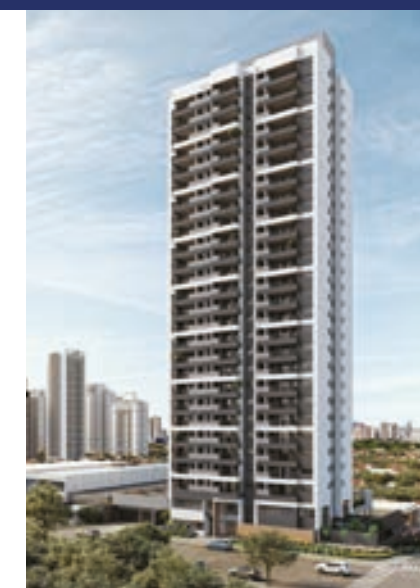
Club Station - Vila Prudente Rua Cavour, 612 x Rua Américo Vespucci Vila Prudente
